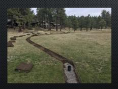
Hole #5, perforated pipe section with "speedy drains" helps to drain approach on par 3
