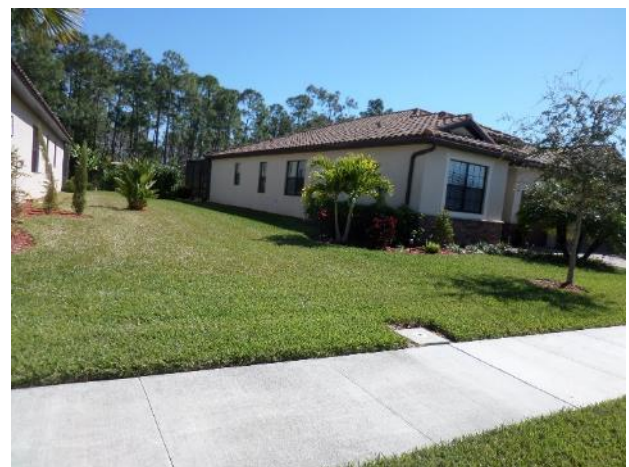
Stains on concrete sidewalk – north area
