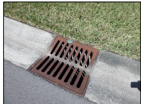
Storm Grate In Good condition
