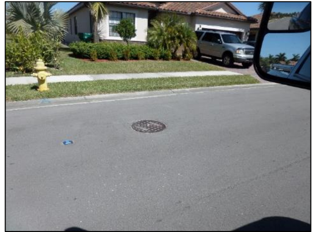
Water stained gutter – south area
