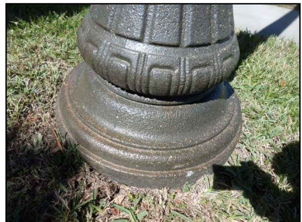
Typical Lamp Post
