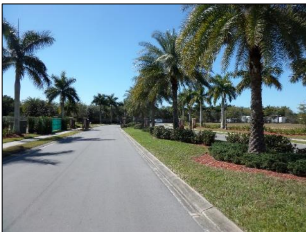
Typical asphalt surface, note water stained gutters-south area
