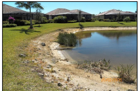
Supply Lines from Submerged Pumps
