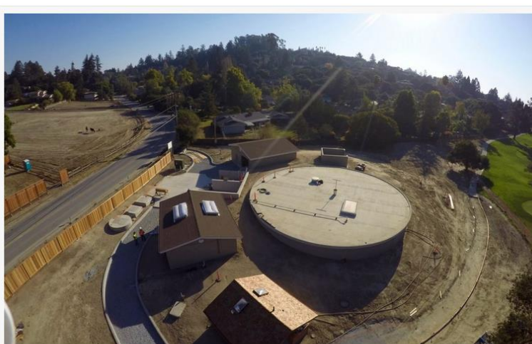
The recycled water treatment facility at Pasatiempo Golf Course in Santa Cruz, California.
