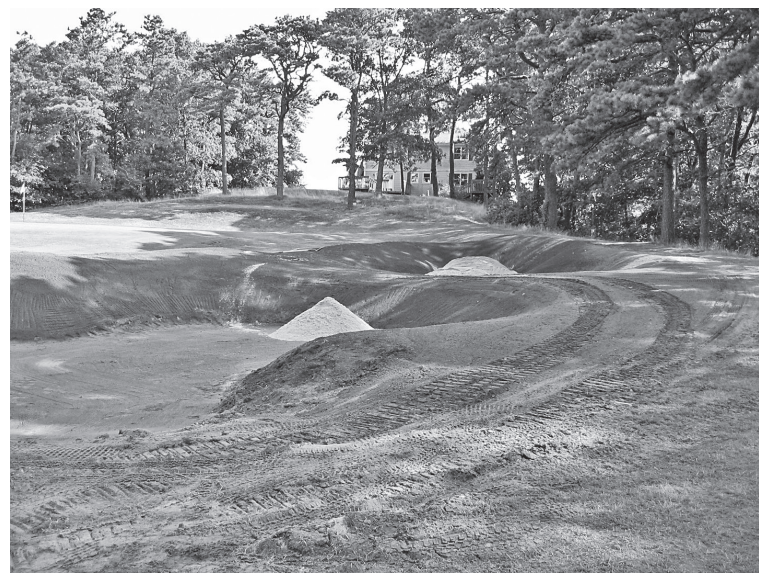
Relocating sand traps to pre-World War II position on Hole 9.
