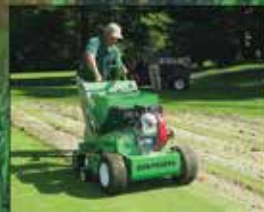
Graden with Sand Injection
