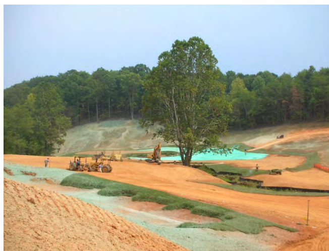
Figure 4. Hydroseeding at Ballyhack.
