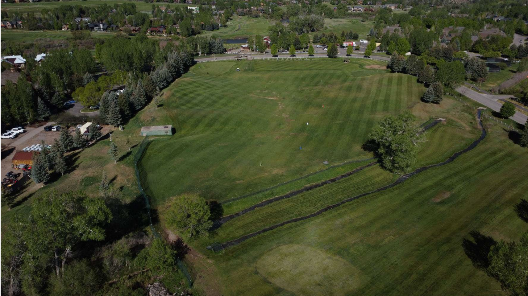
AERIAL VIEW OF POTENTIAL HOTEL SITE
