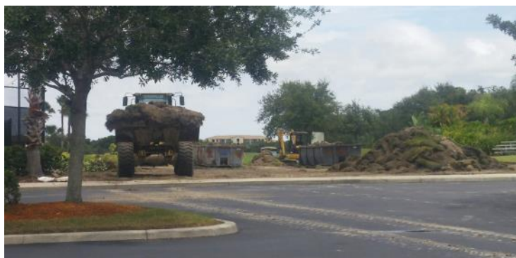
Work began with grass and dirt being removed on August 4th.
