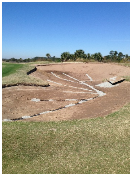
#9 prepped with new drainage
