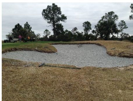
#8 prepped with new drainage and gravel
