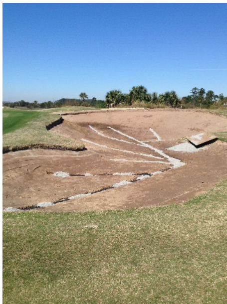
#9 prepped with new drainage
