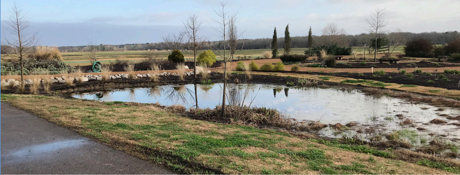
Figure 12. This parking surface drains into a rain garden with unamended soils.
