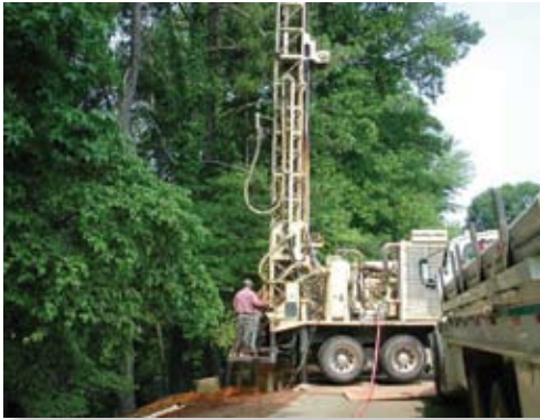
Workers repair a groundwater well at Atlanta CC.
